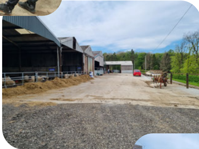
Concrete yard with drainage
